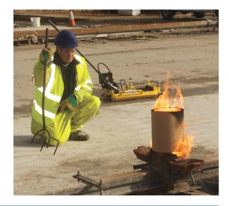
The benefits for continuously welded rail are considerable but they require the rail to be welded on site. Most crane rails are supplied in lengths of 12 metres. Typically rails may be welded into lengths of 300 metres or more with no expansion joint. The rail cross sections are large and the metallurgy; with high carbon and manganese content; make welding difficult.
