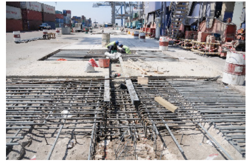
Civil work was completed in sections as illustrated in this photograph
