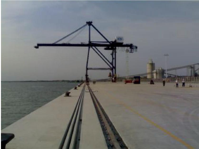
The first of 7 STS cranes of SITV in place at the newly installed Crane Rail System from MHE-Demag Vietnam and Gantrail.
