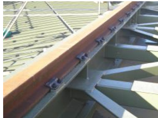
With one rail 'All clips are finally tighten after the rails are welded.'
