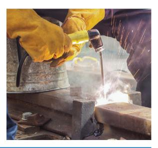
The benefits for continuously welded rail are considerable but they require the rail to be welded on site. Typically rails may be welded into lengths of 300 metres or more with no expansion joint. The rail cross sections are large and the metallurgy; with high carbon and manganese content; make welding difficult.
